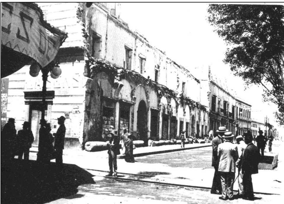
Figure II.15 Demolition of the Carmelites' Portal, 1916
